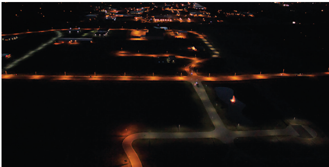
The Portage County Business Park was chosen as a test site for 24 LED streetlights. Half of the lights were installed on the streets in the upper left portion of the photo and the other half were installed on the streets shown at the bottom right.
